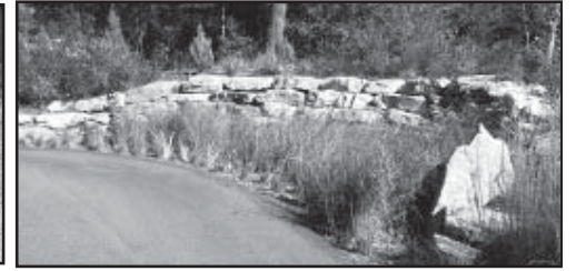
Stormwater bioretention areas often look just like a professional landscaping feature while working to reduce runoff and enhance water quality
