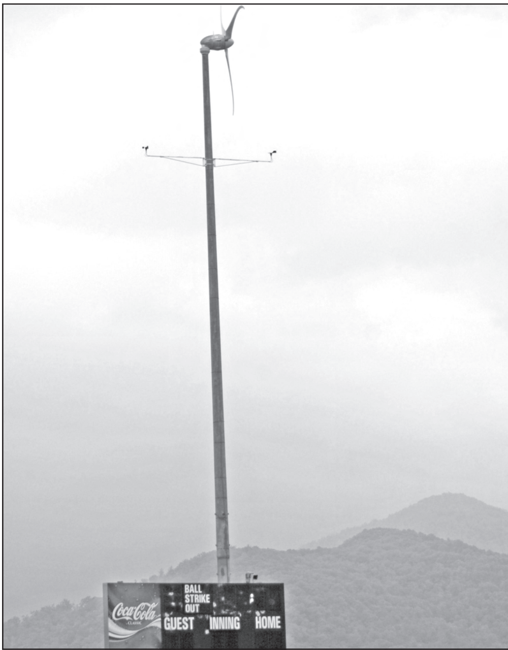
This 60-foot high wind turbine could soon put a dent in the amount of money the school system pays for electricity. The turbine is the first of its kind at a public school in Georgia. Only Lovett, a metro private school, has a similar wind energy project. Photo/Lowell Nicholson
