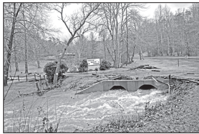
Flooding at Fodder Creek Estates
